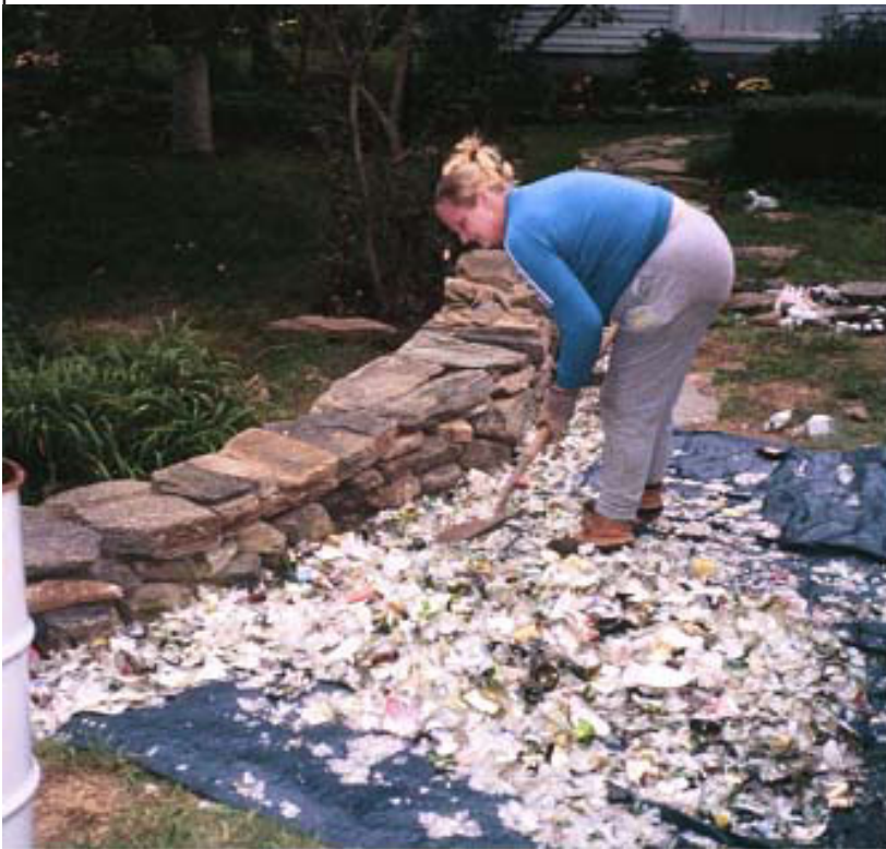
Harpswell resident Megan Hubbard, backfilling her stonewall with recycled crushed glass from the Harpswell Recycling Center
